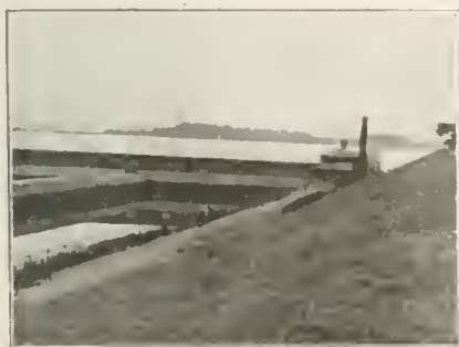
Fig. 1. Collecting tanks and gate house on Moon Island.
